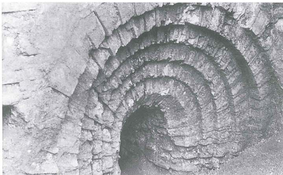
Figure 19. Foundation near Zeyrek Camii.
